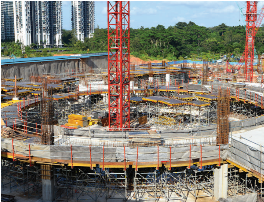
VARIO GT 24 Column Formwork can be adapted to suit every cross section and concreting height.
