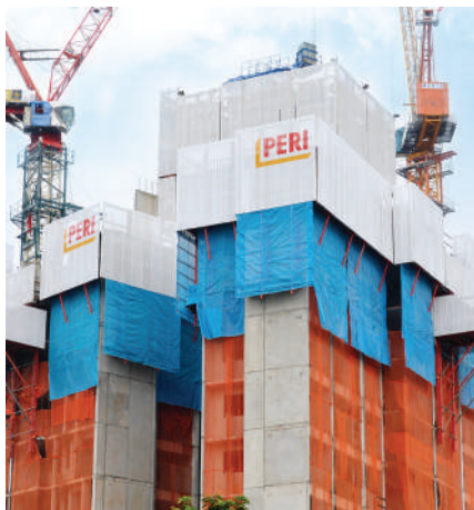
RCS Climbing Platform applied to the 43-Storey condominium.
