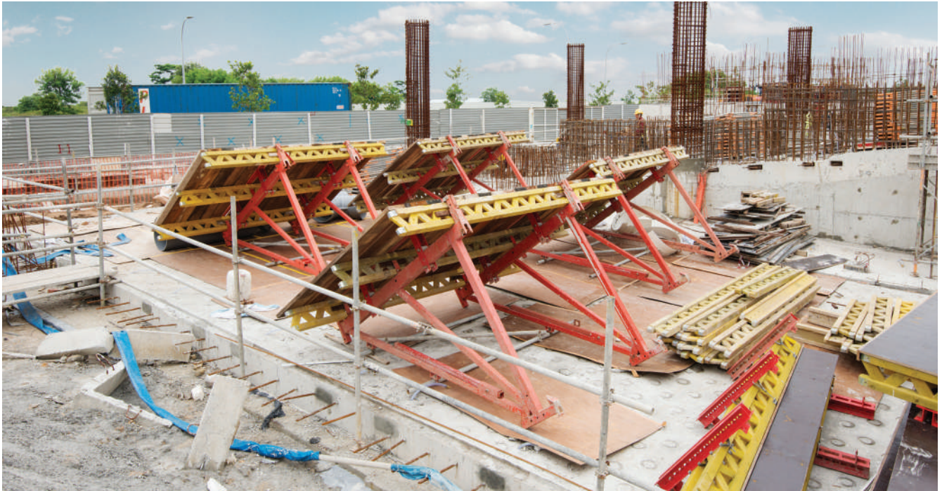
Platforms of CB 240 Climbing Systems.
