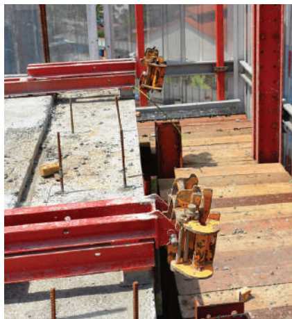
RCS-P provides protection from falling.
