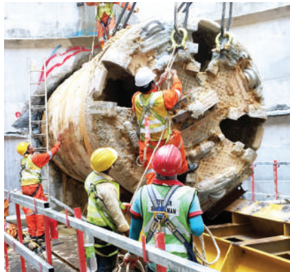
Break through of TBM.
