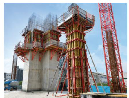
An upclose view of CB 240 Climbing Formwork system in the background and VARIO GT 24 Column Formwork system in the foreground.
