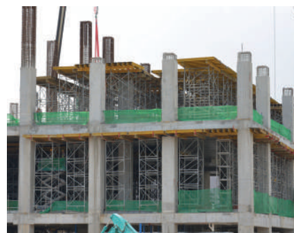
PD 8 Table forms speed up the construction cycle.
