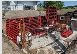
Wall Formwork
